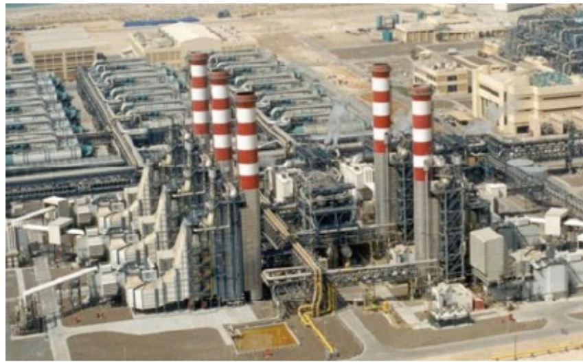
Altauweelah Power Plant, Abu Dhabi, UAE
