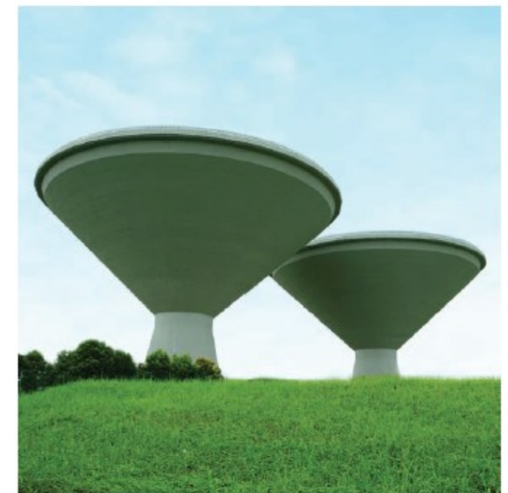
Newater Tanks At Tampines, Singapore
