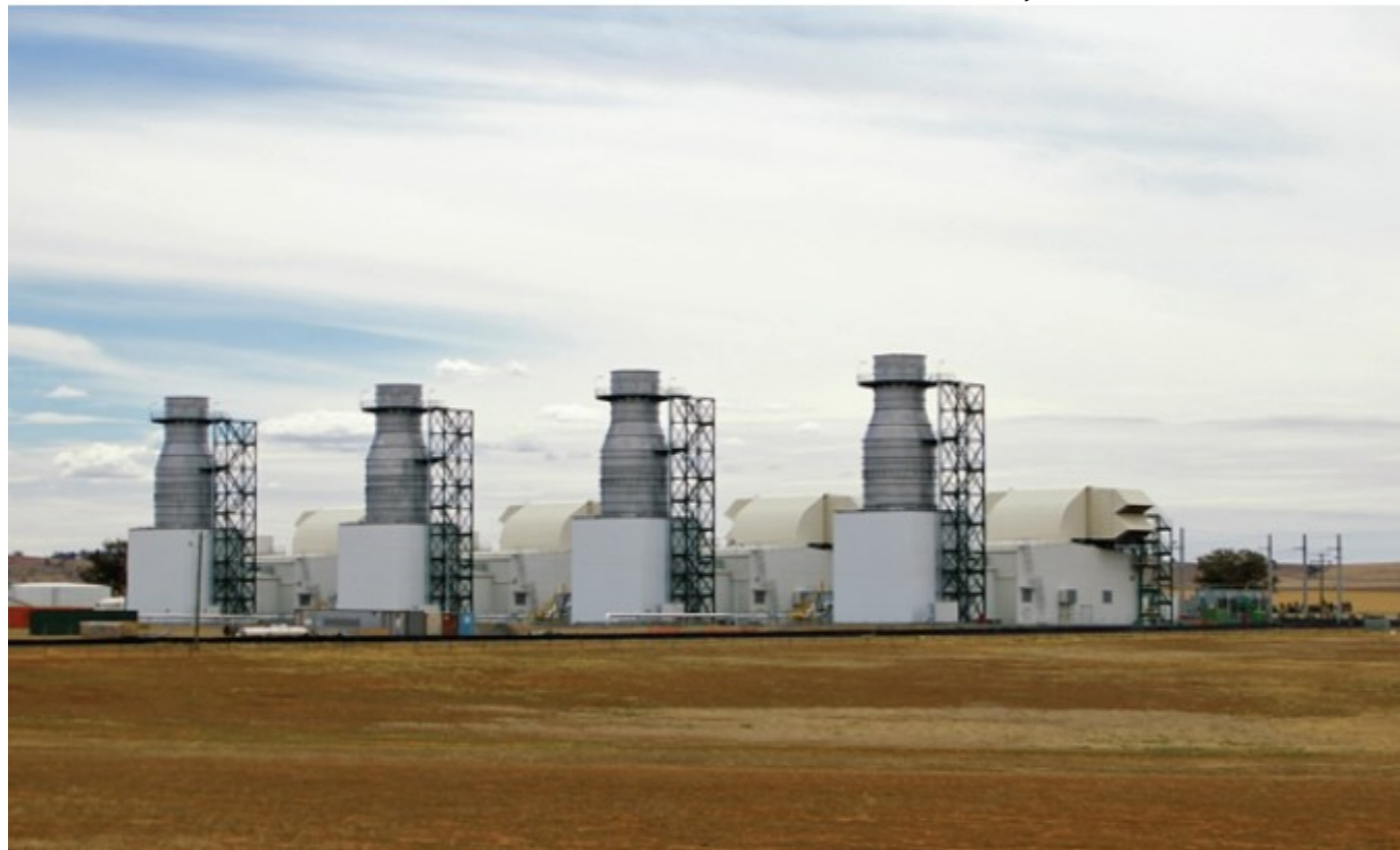
Gas-Fired Electricity Generating Station in New South Wales, Australia
