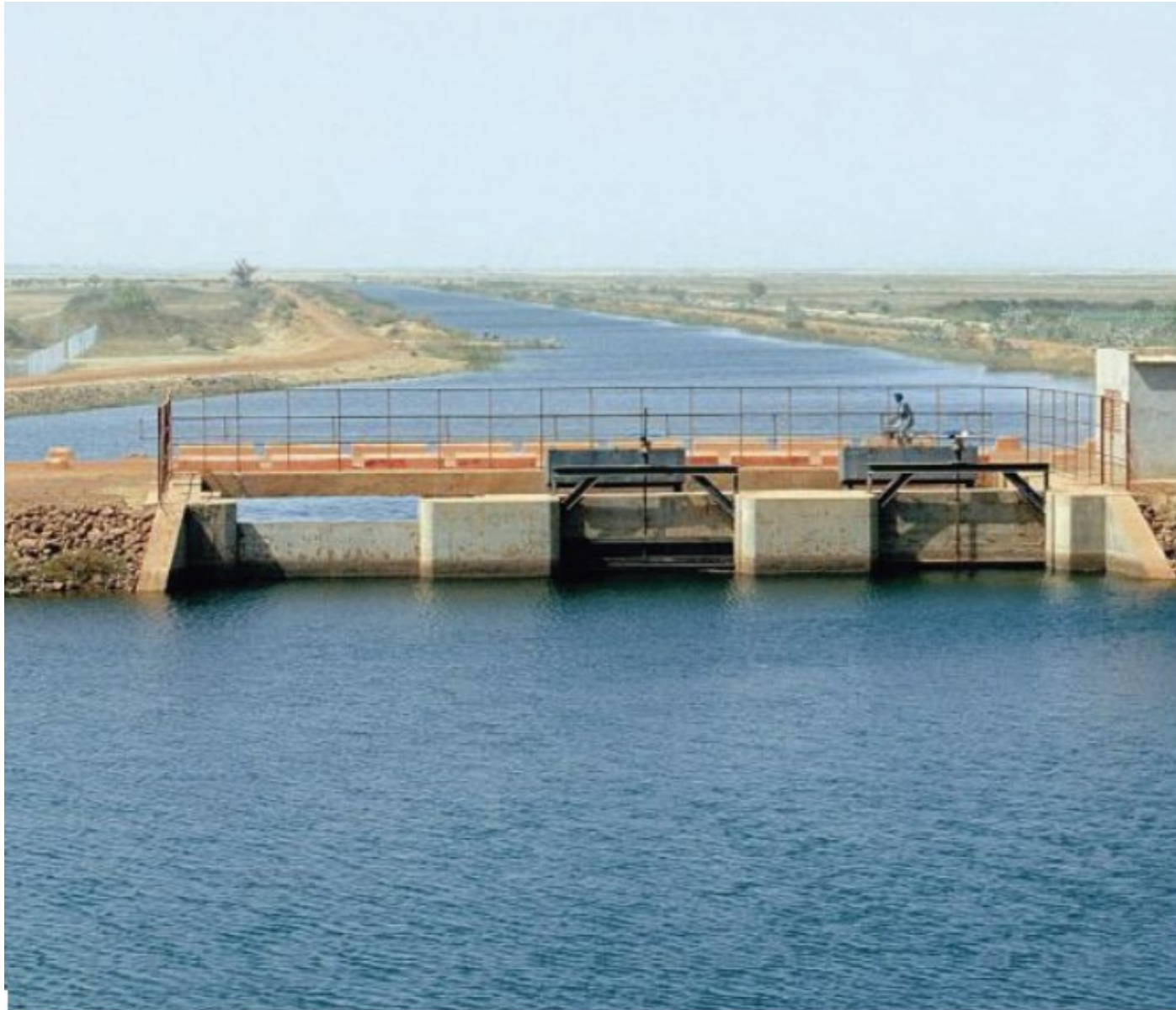
Irrigation and Water Conservancy Project in Siengo, Mali
