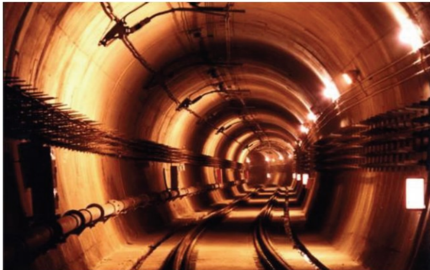
Tunnel of Guangzhou Subway Line 2, China
