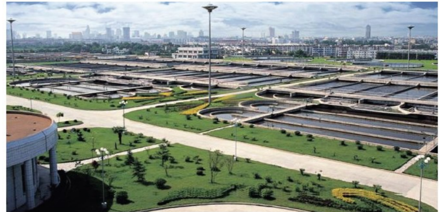
Wangxiaoying Sewage Treatment Plant in Hefei, China
